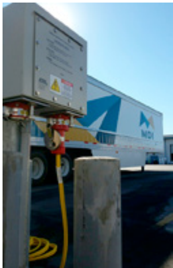
MDI charging station, a Sparx Challenge innovation.
